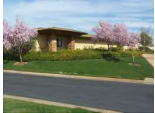
Exterior Surfaces - Typical
