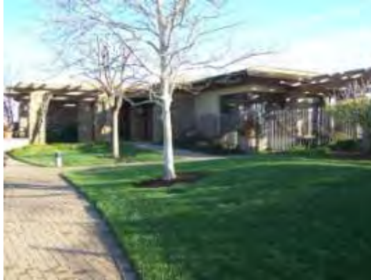
RFS Building Entrance
