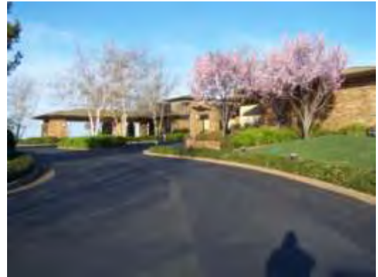
Entrance Drive Asphalt Pavement
