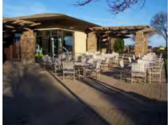
RFS Building Patio
