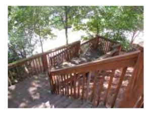
The wood in the exterior stairs expands and contracts with changes in temperature and moisture levels within the wood, leading to cracks. Untreated, these cracks will expand and can lead to the development of rot within the wood.
