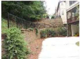
Retaining walls in general are designed to provide slope stabilization and soil retention by means of a structural system. Typically, walls that are three feet high or more require some level of design.
