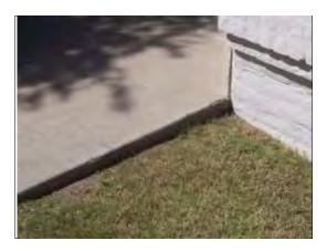
In addition to the concrete work, we found a number of locations where the ground adjacent to the sidewalk is eroded or subsided. We consider these to be a significant tripping and falling hazard. We recommend including this type of regrading and repair work as part of the normal annual grounds contract.
