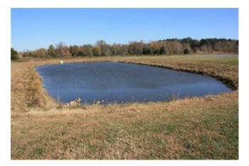
The pond will accumulate silt and over time and lose the ability to store stormwater at design levels, which could result in overflows and minor local flooding. In addition, water quality can be negatively affected by increased siltation and debris accumulation. Accordingly, ponds require periodic dredging.
