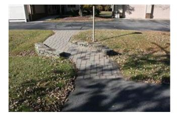
To correct defects and provide the longest service life of the unit paver system, periodic re-setting is required. Re-setting provides an opportunity to replace broken unit pavers, fill in voids in the foundation material, and level the surface areas. We have included an allowance for periodic re-setting of those portions of the system.
