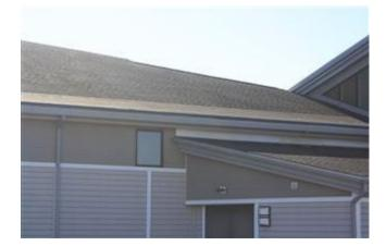
Asphalt shingle roofs can have a useful life of 20 to 50 years depending on the weight and quality of the shingle. Weathered, curled, and missing shingles are all indications that the shingles may be nearing the end of their useful life. The Sanctuary st the Mission was constructed without the proper ventilation nor with an air/water shield at the eves. This situation is currently being corrected.
