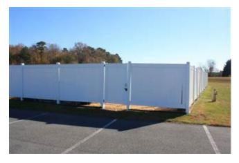
Protection from string machine damage during lawn maintenance can extend the useful life of some fence types. Protection from this type of damage is typically provided by applying herbicides around post bases or installing protective sheathing.
