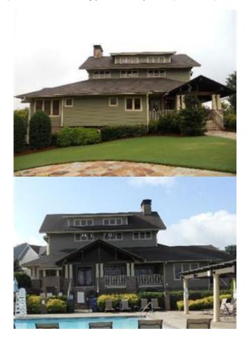
Asphalt shingle roofs can have a useful life of 20 to 50 years depending on the weight and quality of the shingle. Weathered, curled, and missing shingles are all indications that the shingles may be nearing the end of their useful life. Access to the roof was not provided at the time of inspection. Annual inspections are recommended, with cleaning, repair, and mitigation of vegetation performed as needed.
