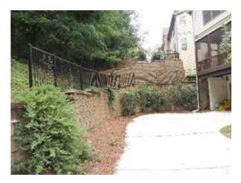
Retaining walls in general are designed to provide slope stabilization and soil retention by means of a structural system. Typically, walls that are three feet high or more require some level of design.
